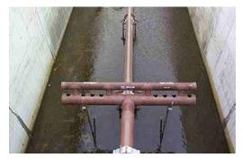
Supernatant Decanters do not include spring loaded valves and liquid can be drawn closer to the surface if needed.
