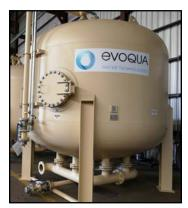
Fabricated vessels meet ASME quality requirements for pressure vessel certification.
