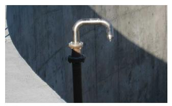
Optional top nozzle for breaking surface crust.
