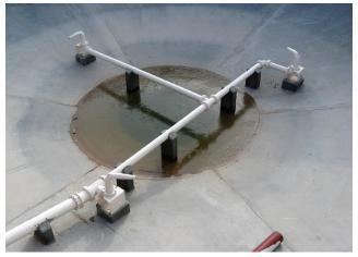
JetMix<sup>™</sup> System proprietary nozzle placement.
