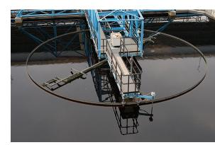
After FEDWA Baffle System settling is improved
