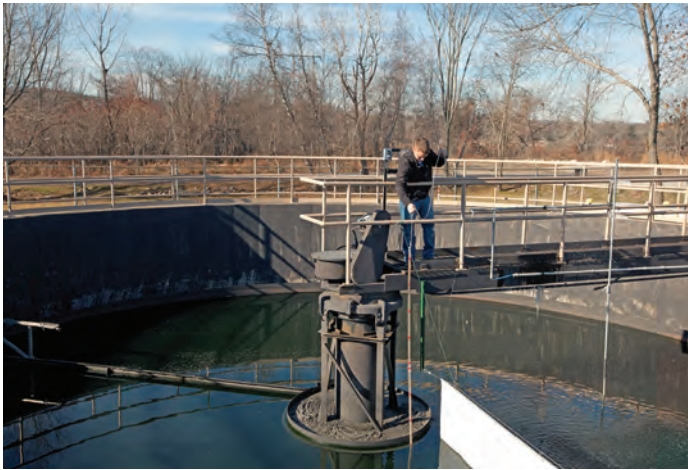
An operator measures the sludge blanket depth in a clarifier. The picture shows no visible signs of sludge buildup or scum in the clarifier.
