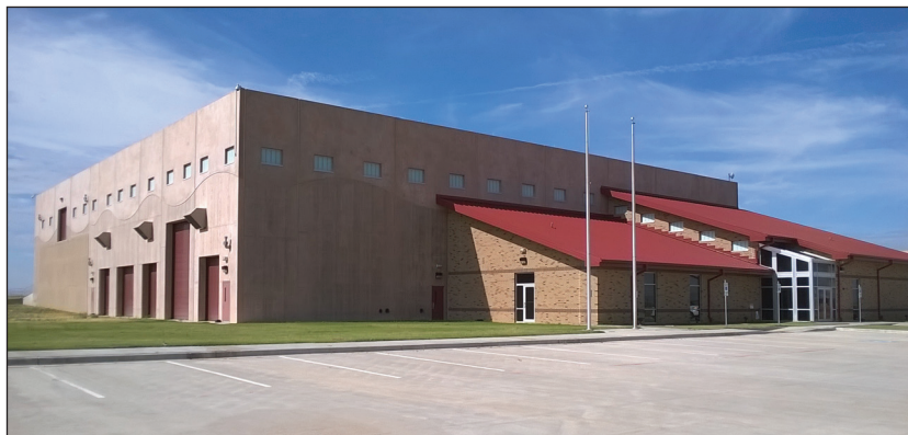
The 15 mgd South Water Treatment Plant in Lubbock, Tex., came on line in 2012. Photo courtesy of the City of Lubbock, Tex.
