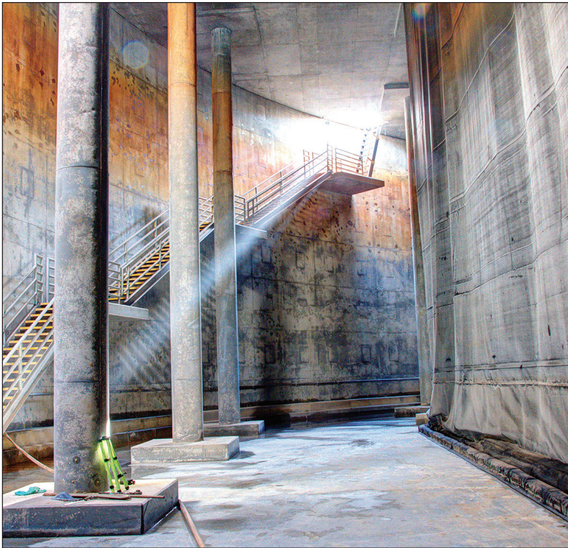
The West Clearwell serves San Diego's 34 mgd Otay Water Treatment Plant. Photo by Jim McVeigh, City of San Diego, Calif.
