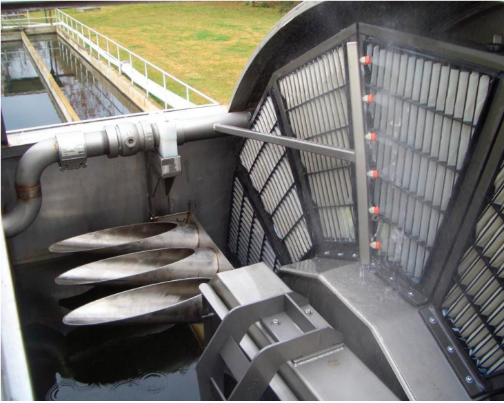
The spray mechanism is specifically designed to efficiently release solids from the pleated media.
