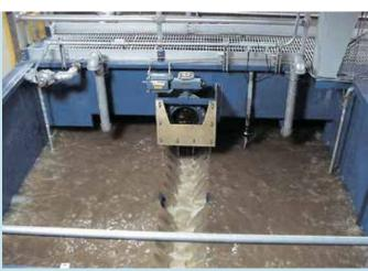
Backwash water flowing in trough, air assisted
