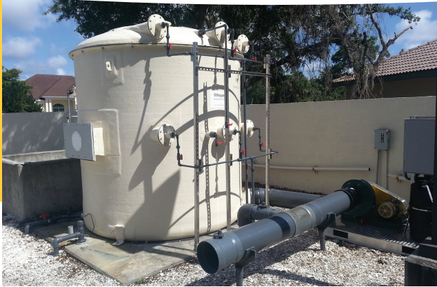
WHISPER® Biofilter System
