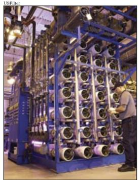
**FIGURE 3.** Reverse osmosis membranes can be cleaned onsite or off-site, depending on your facility's needs. Auditing membrane condition on a regular basis can alert you to other issues within your water-treatment system
